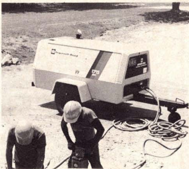
A Spiro-flo portable compressor in action.
